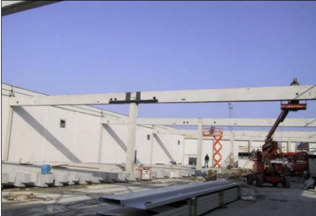
**Figure M12.4:** Overview of the hybrid strengthening work
