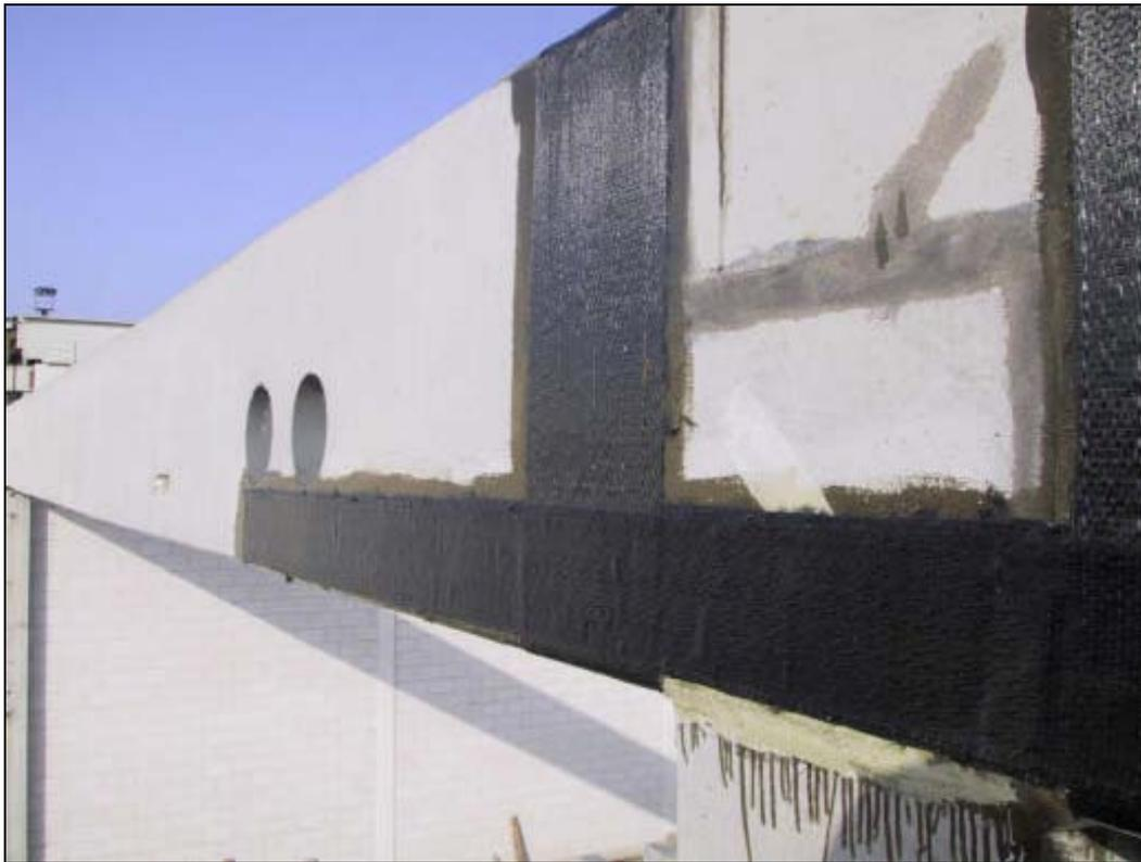
**Figure M12.5:** Detail of the connection of the two beams, showing epoxy mortar filling of original joint between beams, and continuity reinforcement above middle support
